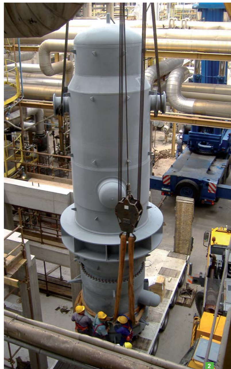
2 HP Steam Superheater, 2.25 Cr alloy, Jacobs - Yara, Ferrara Italy
