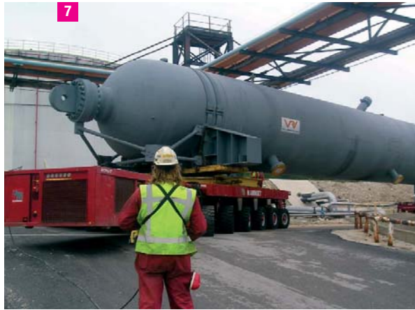
8 C2 Hydrogenation Reactor, 1.25 Cr alloy, Technip - Yanbu National Petrochemical Co., Yanbu refinery, Saudi Arabia
